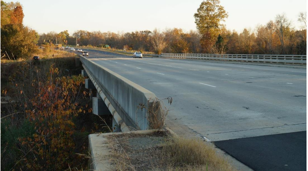
Figure 22: NC 54 Bridge over the Haw River
