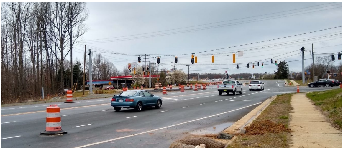
Figure 57: Roadway Improvements under Construction in Mebane
